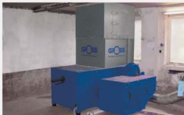
GAZ 102 set up below ground, with hopper expansion
